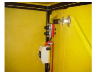
Provision for electrical connections
